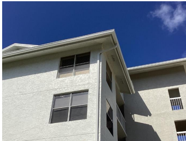
Aluminum gutters and downspouts
