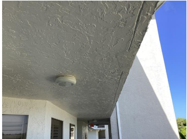
Previous repair at breezeway underside
