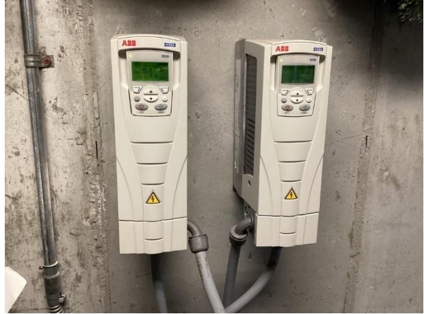
Domestic water pump controls
