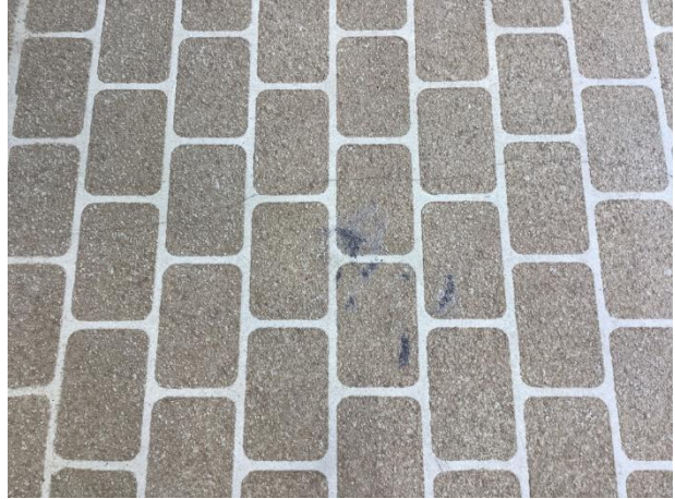
Coating deterioration
