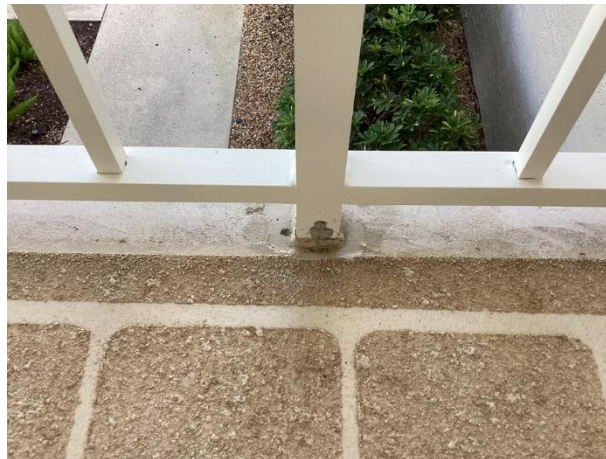
Previous repair at post pocket
