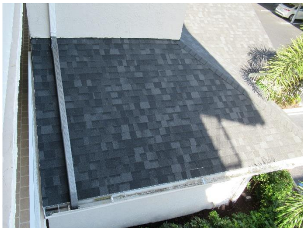
Asphalt shingle roof
