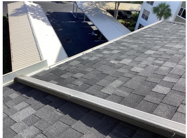
Aluminum gutters and downspouts
