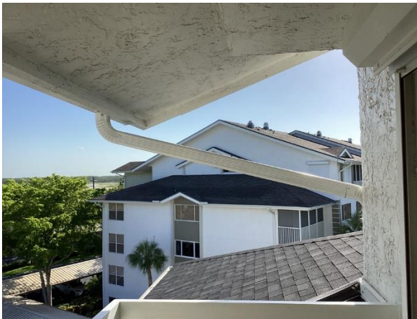
Aluminum gutters and downspouts
