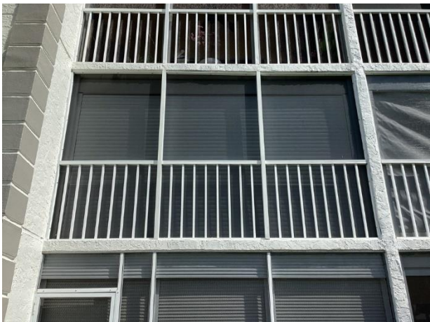
Aluminum railings and screen enclosure
