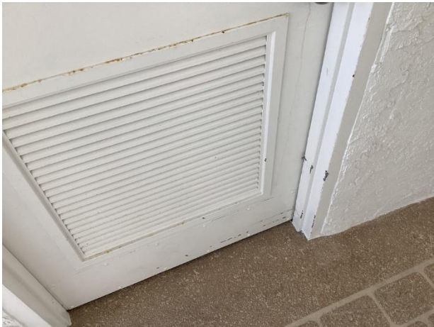
Minor rust at exterior door
