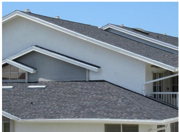
Asphalt shingle roof
