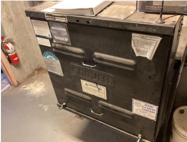
Hydraulic elevator equipment
