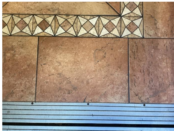
Tile cracks
